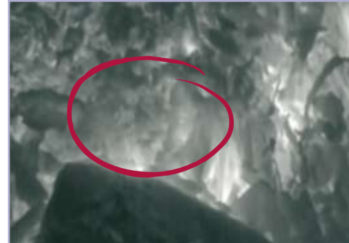
Gas leak on land fill surface
